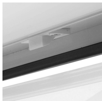
Pull-in blocks ensure tight compression of the sash gaskets against the frame.
